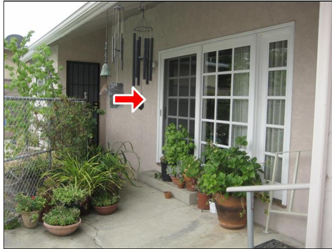
2.1 Item 2(Picture) Rear sliding door
