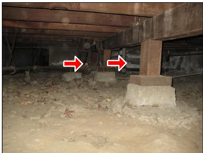
5.2 Item 1(Picture) Piers
