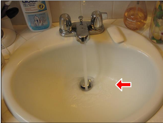
6.0 Item 1(Picture) Non restricted drain
