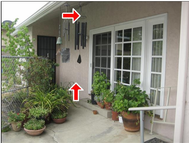
2.0 Item 1(Picture) Stucco walls
