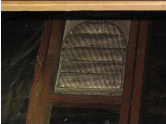
9.3 Item 1(Picture) Gable end vents
