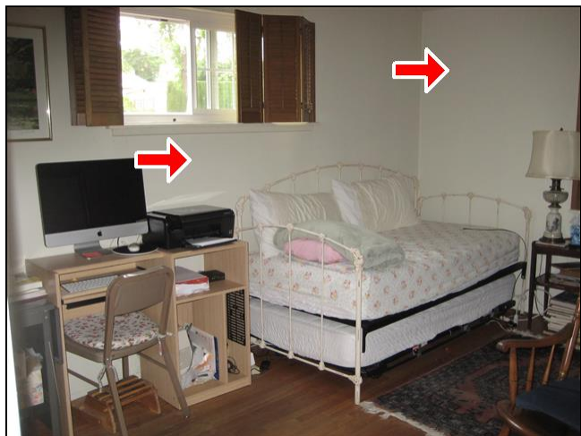
5.1 Item 1(Picture) Structural walls not visible
