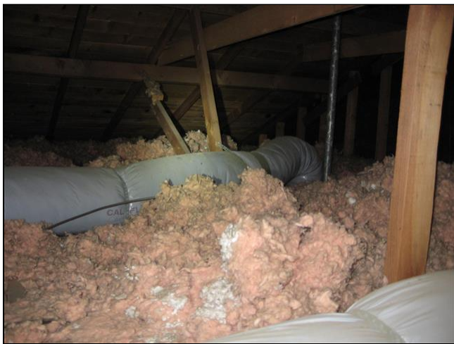
9.0 Item 1(Picture) Insulation
