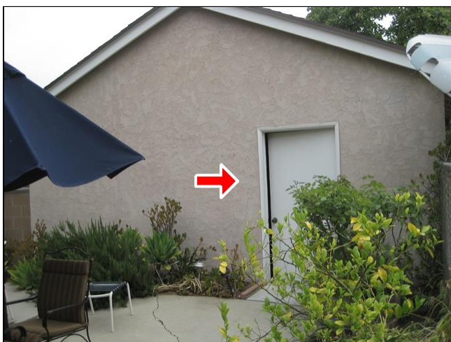
3.3 Item 3(Picture) Passage door
