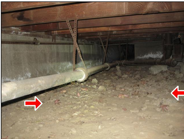
9.3 Item 3(Picture) Dry crawlspace
