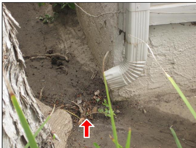
1.3 Item 1(Picture) Gutter Elbow
