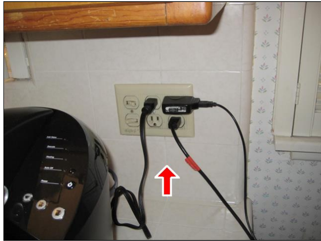
7.4 Item 2(Picture) Kitchen Outlets
