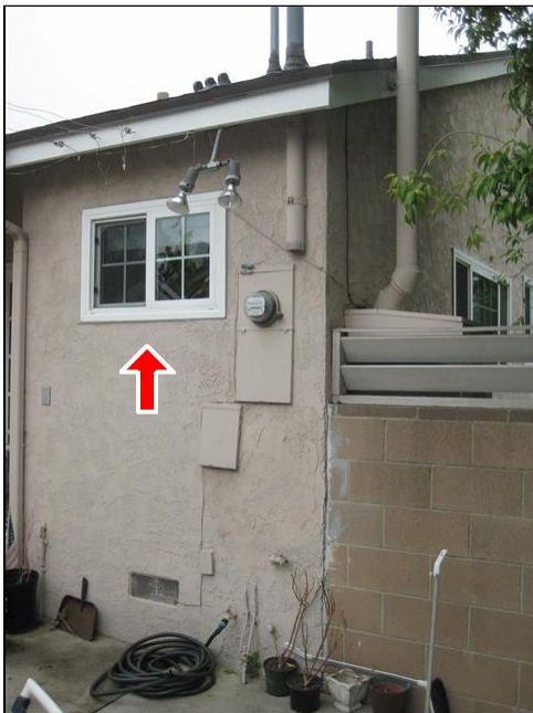
2.2 Item 1(Picture) Window exterior
