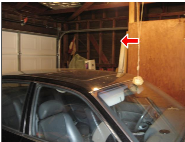
5.1 Item 2(Picture) 2 X 4 construction
