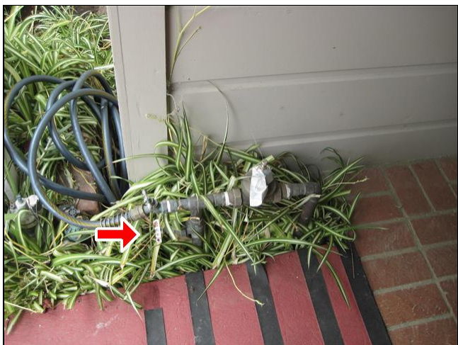
6.3 Item 1(Picture) Main water shutoff
