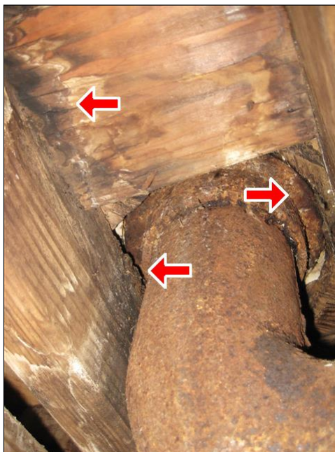
5.3 Item 3(Picture) Master Bathroom Toilet
