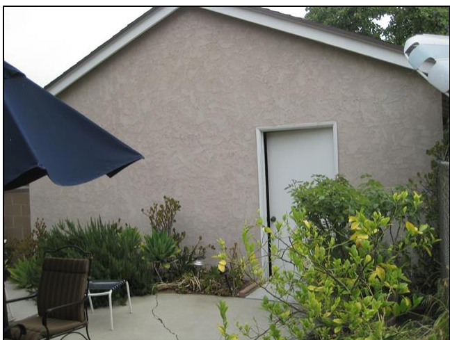
3.1 Item 1(Picture) Detached garage
